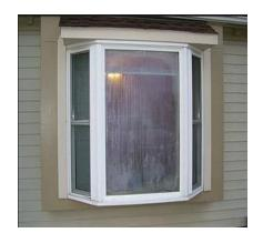
Windows with double pane thermal glass units/glazing in most newer homes and replacement windows in older homes have a tendency for the thermal seal to break between the two panes of glass. When the seal is compromised, air is allowed to enter between the panes which causes condensation and discoloration. This may be easy to detect or it may go completely undetected until these obvious signs occur. In many cases, the first time it will be noticed is when outside temperatures fluctuate greatly.
