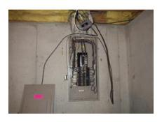
It is common for homeowners to finish their basements to create more living space. If not done by an electrician there could be issues that arise. The most obvious concerns are open electrical work boxes and wiring terminations outside of electrical work boxes. When a sub panel has been added multiple issues can arise. Sub panels are unique on isolation of neutrals and grounds and the way the panel is bonded.
