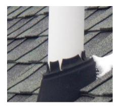
Penetrations at the plumbing vents (roof jacks). The rubber flashing commonly fail as soon as 7 years due to the sun's UV rays breaking them down, and are sometimes split or damaged at installation. When the flashing fails, water can enter through the roof penetration, though it may take some time before the stain is visible. The best practice is to inspect these from the roof surface since the damaged rubber flashing commonly splits on the high side, which is unable to be seen from the ground.
